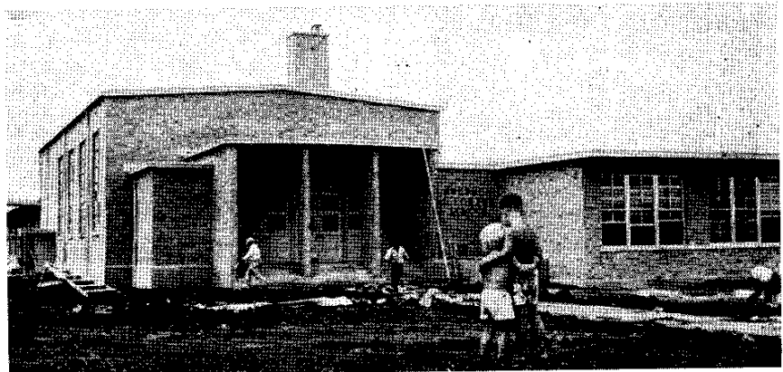
NEWEST IN DALLAS , the Stephen C. Foster Elementary School was completed in August and is ready for final inspection by the Board of Education. The major unit cost $525,043.
